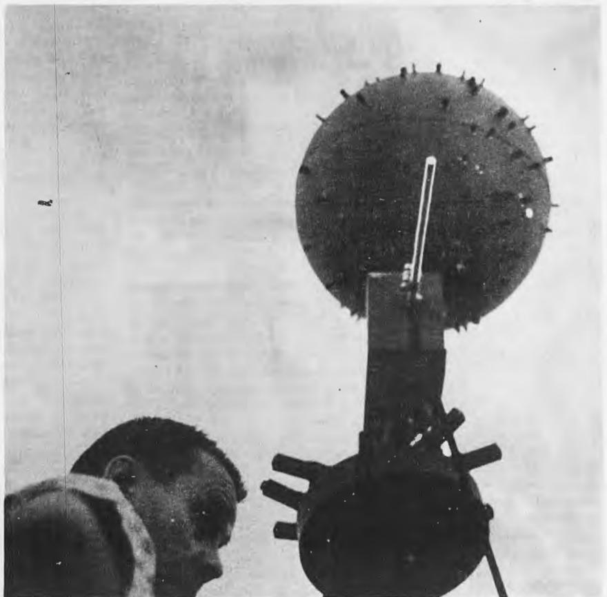
The stars are projected through small holes and lenses in this sphere and are displayed on the dome above.
