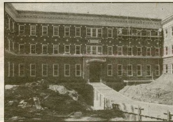
Remodeling project at Sutton Hall
