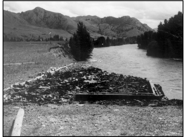
The remains of the loft after the flood. (Courtesy Ed Summerfield)
