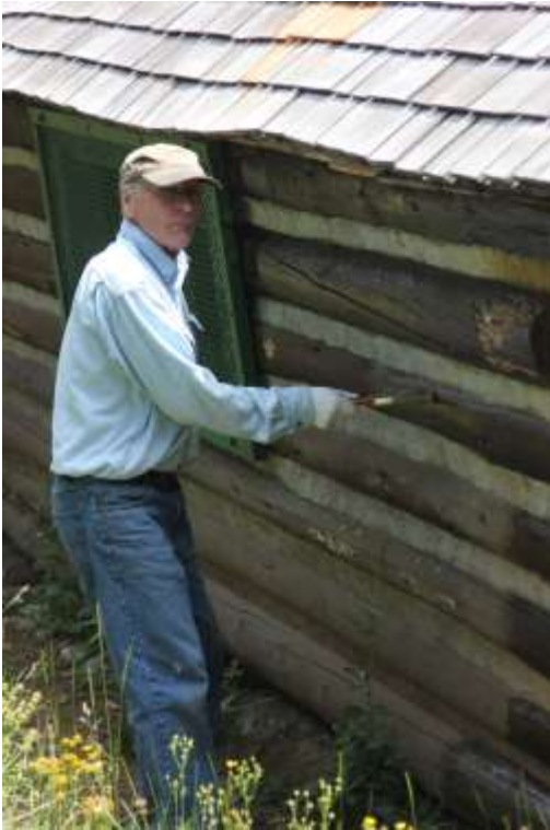
Dave applying oil to the cabin wall.
