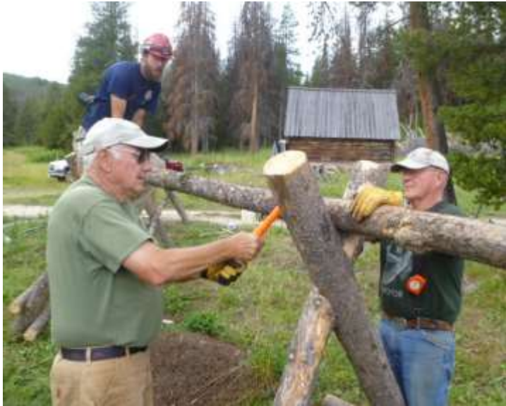
Spiking a rail to Jack-leg. Front L to R: Chuck Fricke, Jack Atkins Back: Sean
