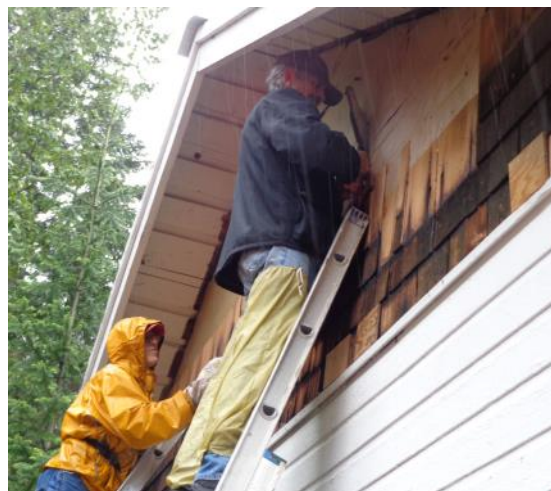
Hank and Rich removing shingles.
