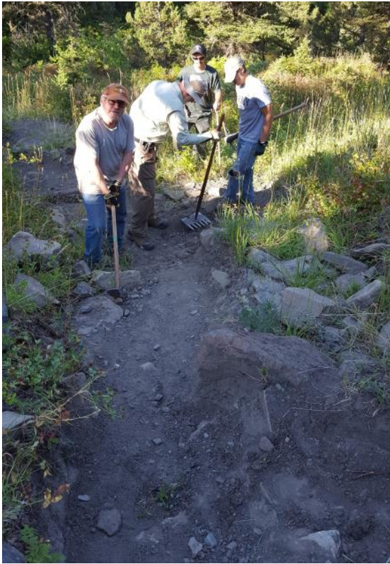
John, Lonetree, Fred working on the trail.
