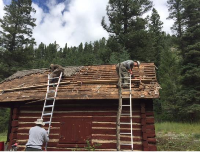
Mark and Alan removing the old roof.
