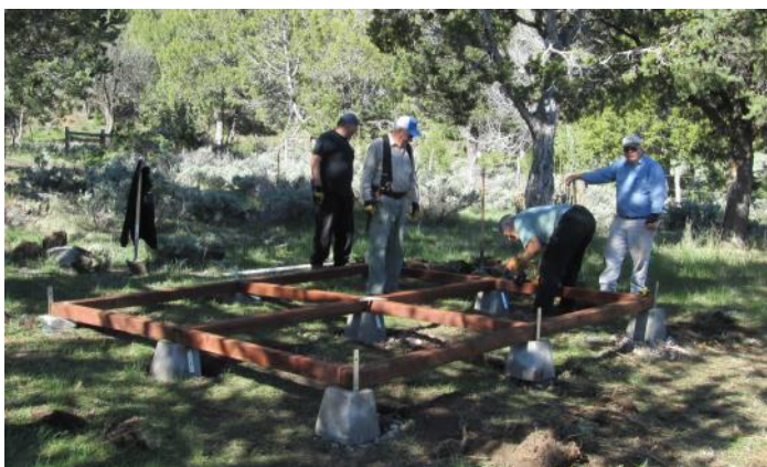
Laying the framework.
