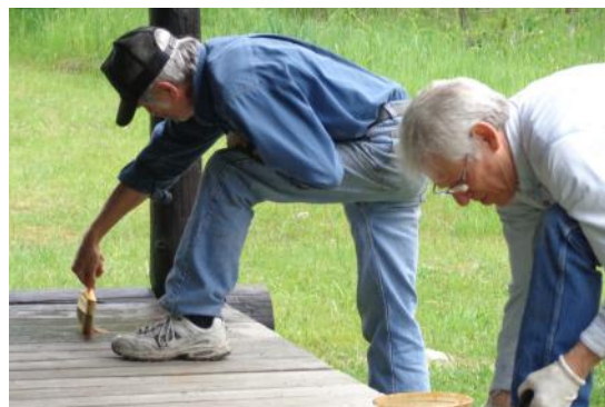
Hank Jones and Rich Appis apply preservative stain to log cabins.
