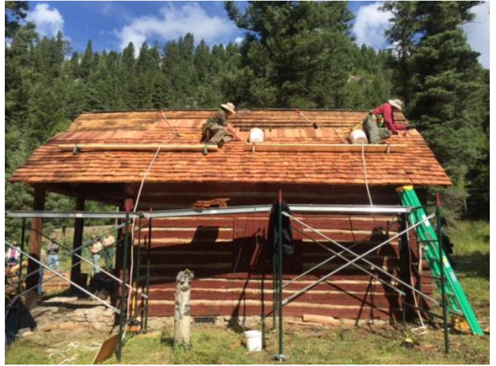
Mark and Bob putting the new shingles on.
