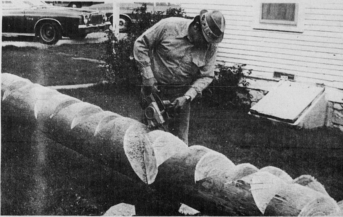
THE MAIN CUTS AND NOTCHES are made by using the larger of Paul's two chain saws.
